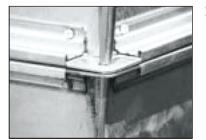
15. Carefully align mating frames before they touch. Ductmate 440 adheres on contact. A drift pin can be used to correct misalignment
