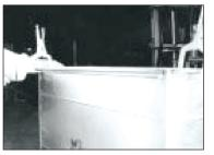
9. Work in one direction around duct when seating the frame. Fasten in sequence as you go. Do not fasten angle at corners first, it can cause seating problems.
