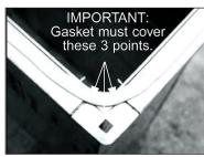
12. Position 440 Gasket in an arc so that it covers the three points in the duct corner. Gasket must cover all three points. Some gasket will protrude into the airstream. Press gasket firmly into contact with the raw edge of the duct corner and WDCI corner assembly. In steps 11, 12, 13, and 14 Ductmate 440 is the preferred gasket. Ductmate Neoprene Gasket may be used where a section must be disassembled.
