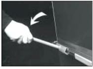
17. WDCI cleat can be snappedon with the Snapper I Tool or with the Snapper II where space is restricted.
