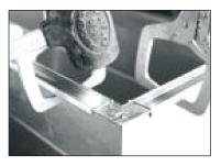
7. Use a mallet to seat the frame onto the duct.
