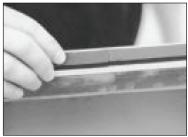
4. Apply Neoprene gasket completely around WDCI frame to the beginning point. Butt the two ends of the gasket up against each other. Do not overlap the two ends.
