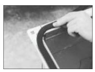
Position Neoprene gasket in an arc so that it covers the three points in the duct corner. Gasket must cover all three points.
