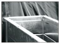
11. Start approximately in the middle of one side, place a single strip of gasket tape completely around the inside edge of the angle frame. At the corners, the gasket must cover the exposed edge of the duct section and the gap between the duct wall and the WDCI corners.
