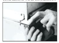
16. Insert a 3/8" x 1" nut and bolt for WDCI J Connection Systems.
